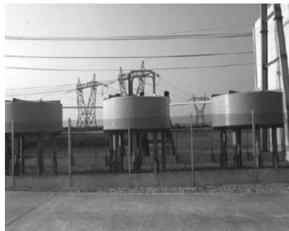
Figure 10. 20-kV, 20-MVA (per phase) dry-type, air core, tertiary-connection shunt reactors.
